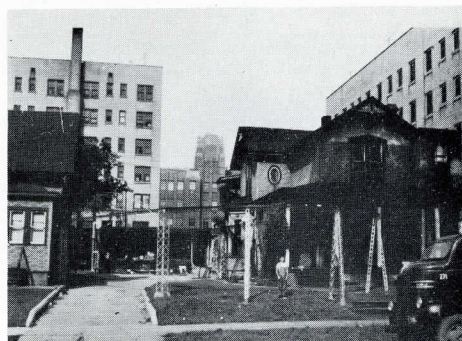
Front View Showing Trestle Leading to Swedish Bridge
