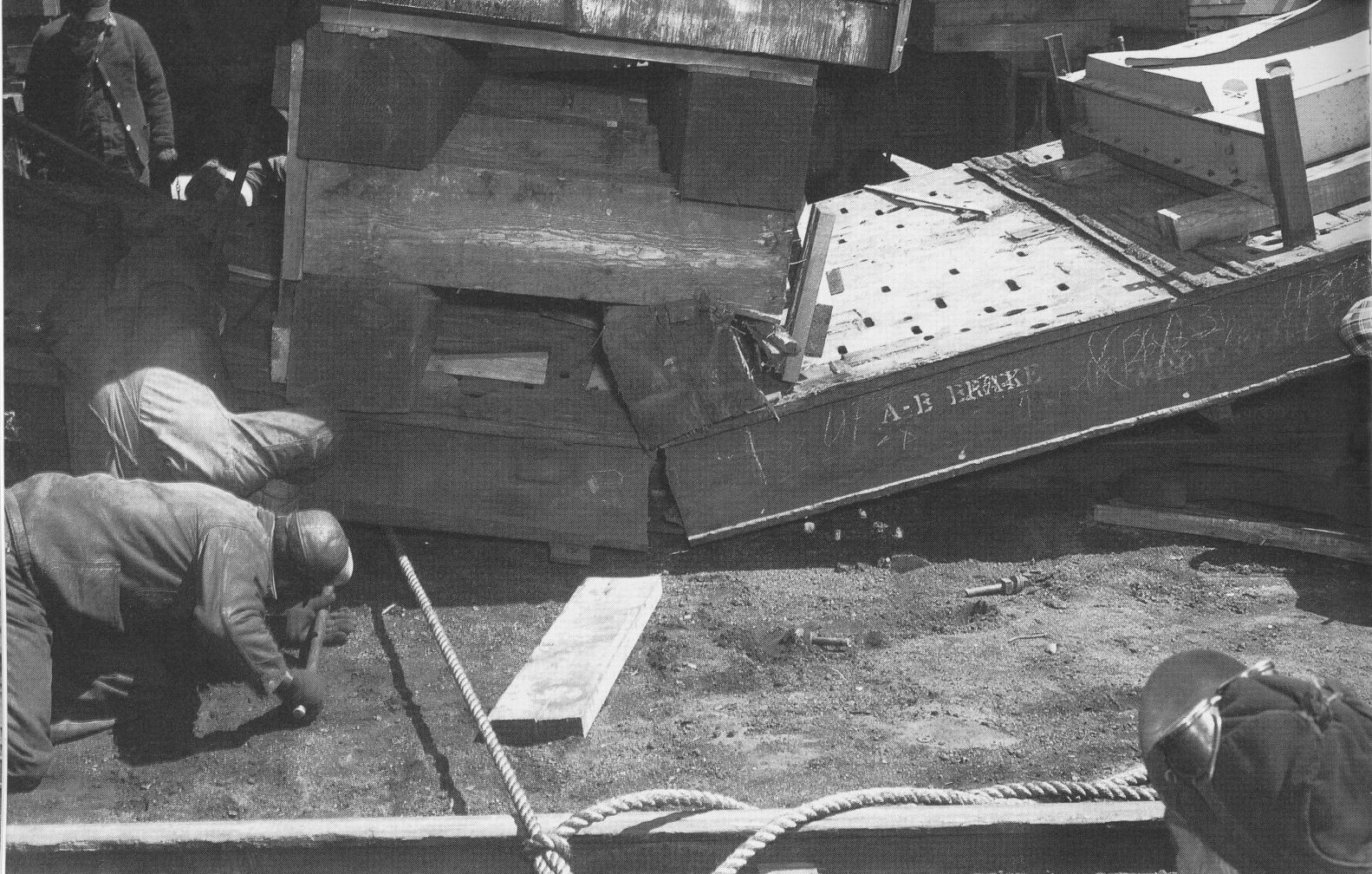
Above: A rescue crew begins the difficult task of recovering broken flat car 48053. The ropes and pry bars are the first assault on the car — a crane is undoubtedly already on the way out to help pick up the broken pieces. Note that by this time the car has been updated to have AB brakes. —C&NWHs Archives
